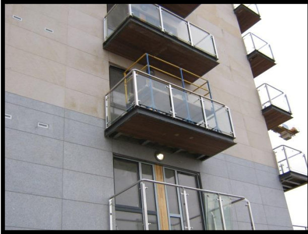
Balcony Soffit Cladding (John Fleming Construction, Dublin)
