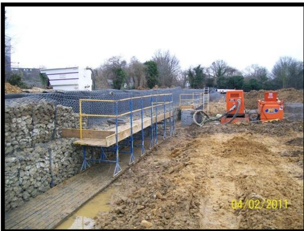
Installation of Gabion Walls (C.A Blackwell - Balfour Beatty – London)
