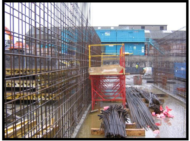
Steel fixing (Daninger Construction Ltd)
