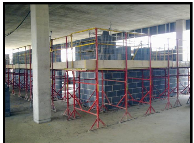
Blockwork (C& I Smith - Wates - Wakefield)
