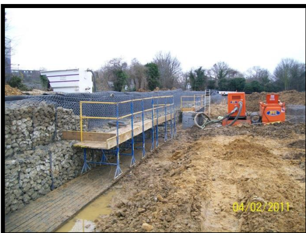
Installation of Gabion Walls (C.A Blackwell - Balfour Beatty - London)
