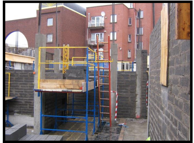
Blocklaying (BAM Construction Ltd)
