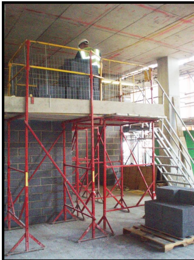
Pacebrow Brickwork Ltd – BAM – West London
