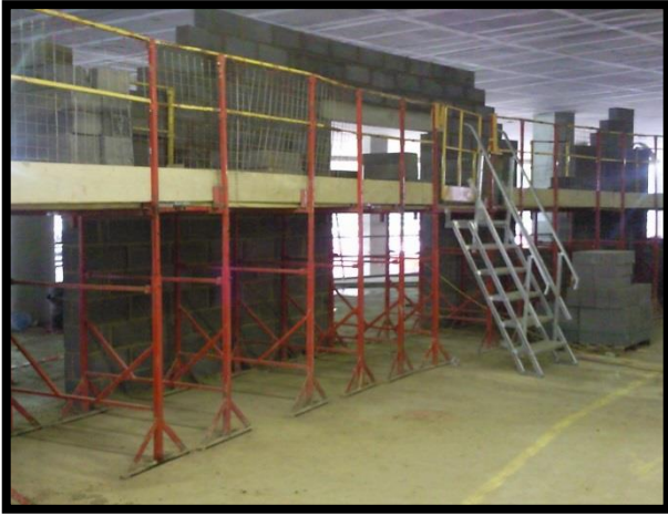
SafeStand® 1200's On a Curve (Laing O'Rourke at Pembury Hospital)
