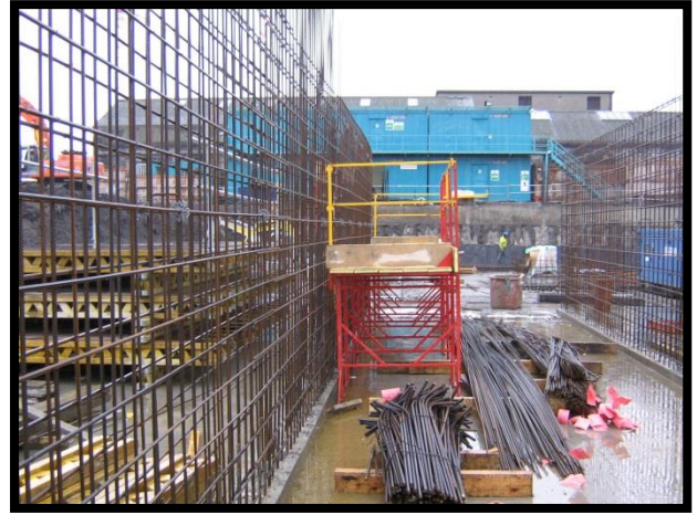
Steel fixing (Daninger Construction Ltd)
